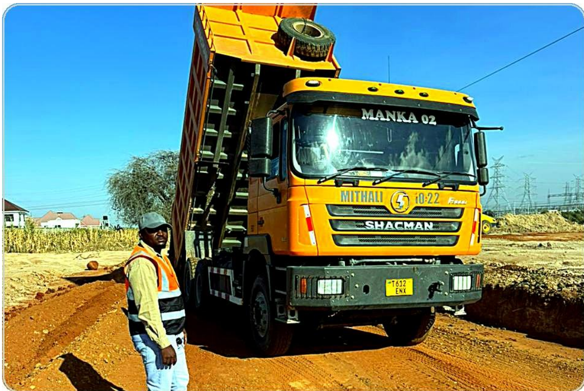
Delivering and placing material on site with our tipper fleet.
