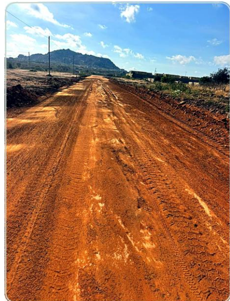
A graded road surface was completed by our team.
