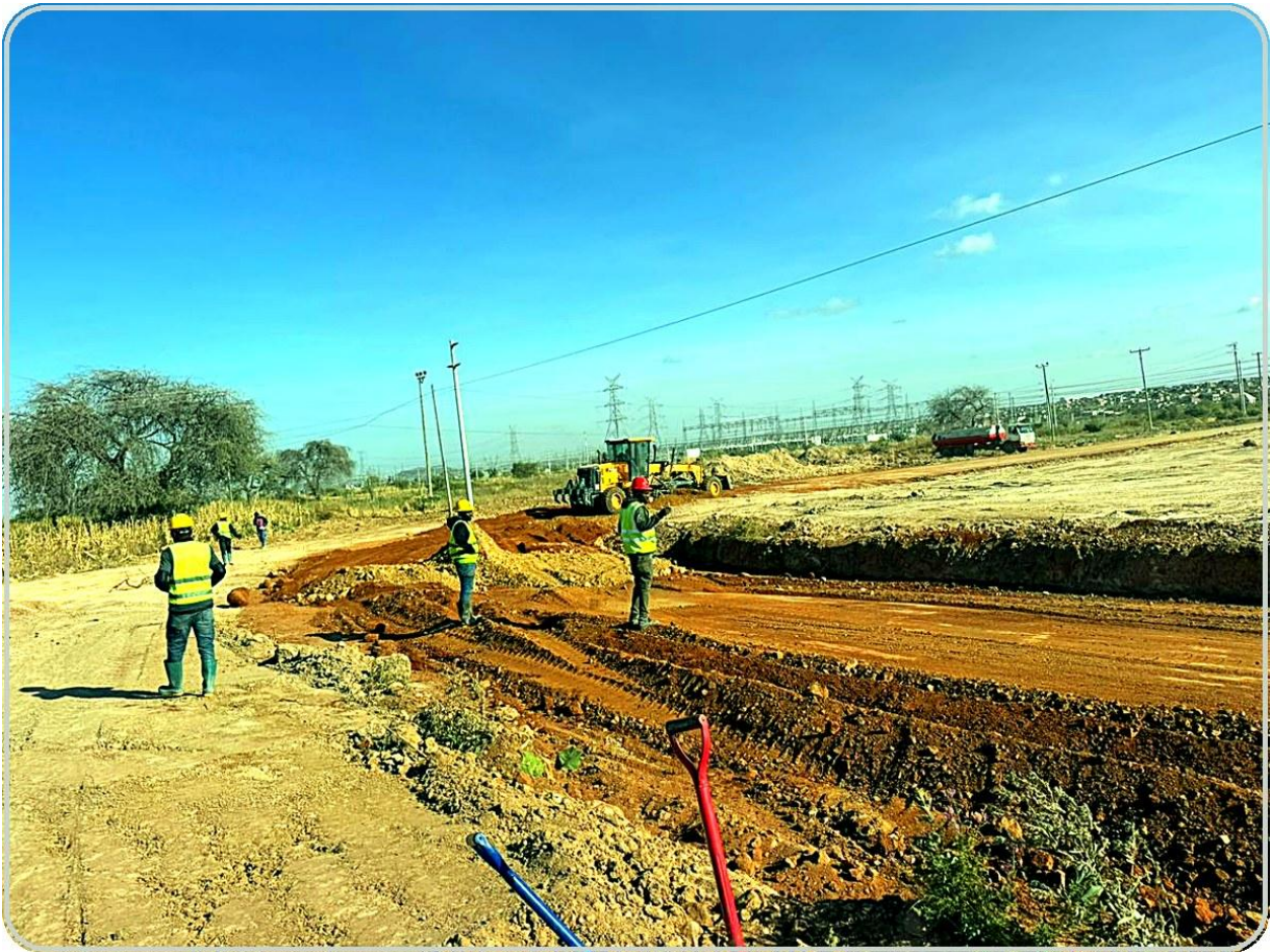
Our site team supervising works in progress.
