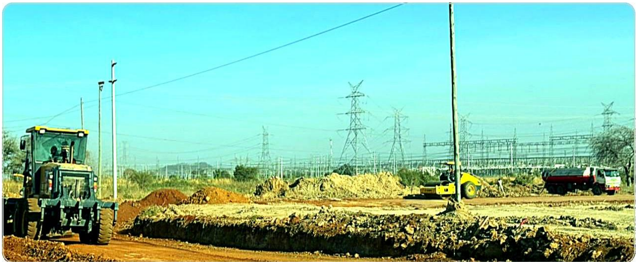
Our equipment and team at work on an active road construction and earthworks site.
