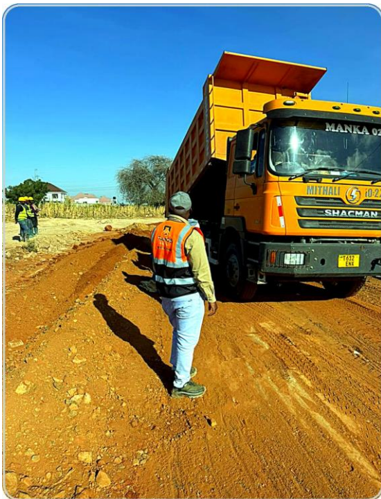
Offloading and placing material on site.
