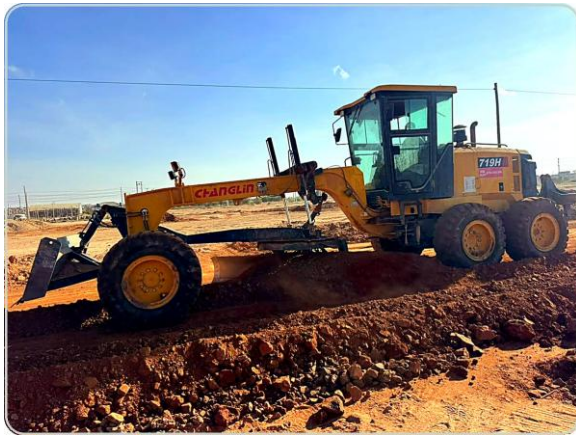
Motor grader shaping the road formation.
