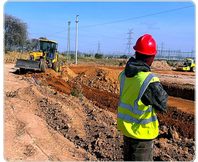
Grading and compaction work underway.
