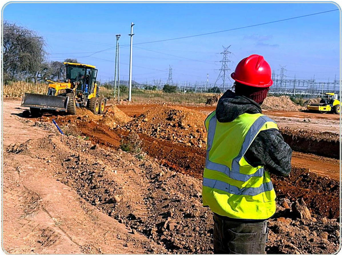
Safety first, our team is on site in full personal protective equipment.
